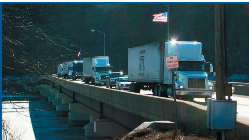
Trucks on the Blue Hill Bridge, waiting to enter Northumberland...
