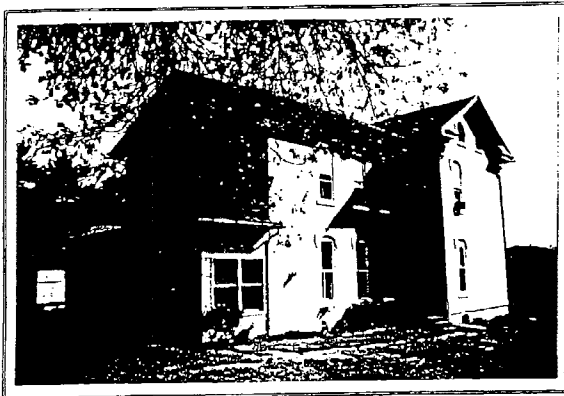
Mertz Family Historic District (220): Photo 2 - View of north and east (rear) sides of brick Italianate house. The first house on the property purchased by the Mertz family in 1906 is adorned with segmental lintels and decorative cornice brackets.
