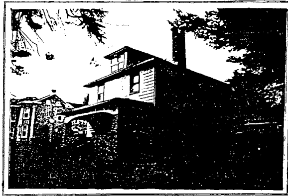
Mertz Family Historic District (220): Photo 6 - View of west (main) and south facades of the fully intact foursquare house. Note the Craftsman style porch. The house was built by William Henry Mertz, Jr. during a period of growth for the family greenhouse enterprise.
