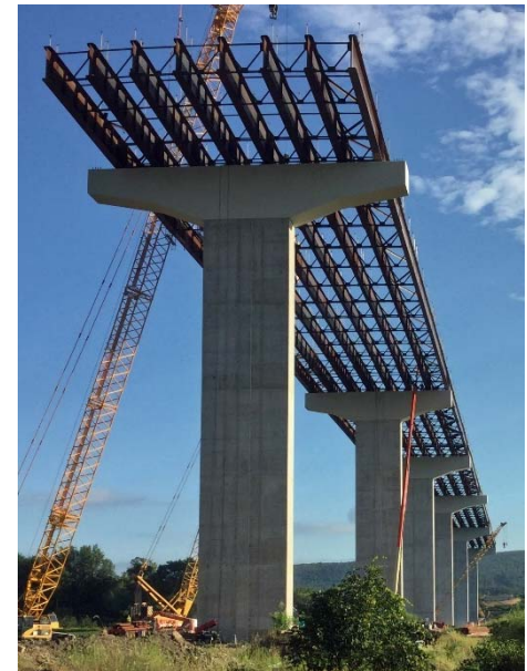
CSV T River Bridge Construction (looking northeast)
