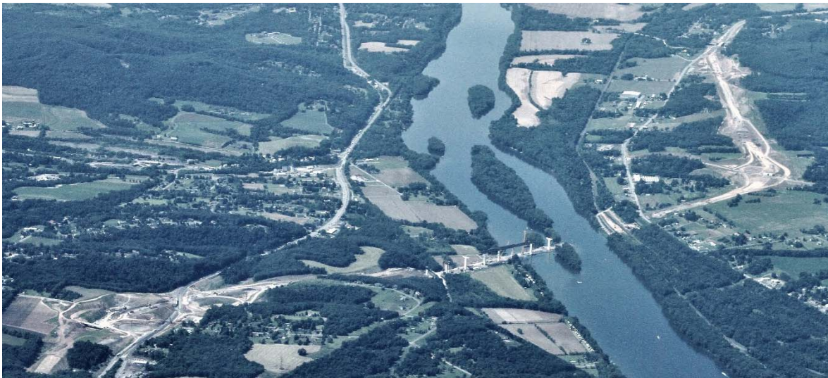
CSV T Northern Section Construction (looking north)
