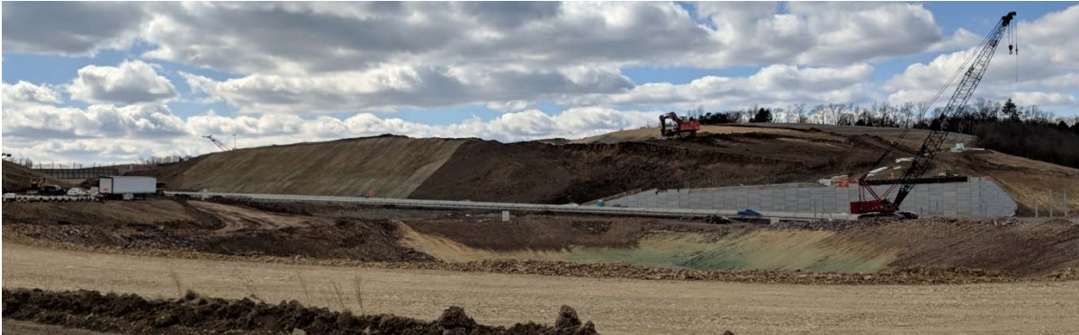
US 15 Interchange Construction (looking southwest across US 15)
