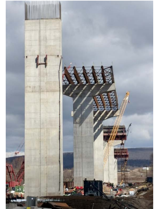
CSVT River Bridge Construction (looking northeast across river)
