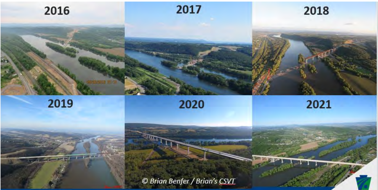
Yearly progress of the river bridge construction.
