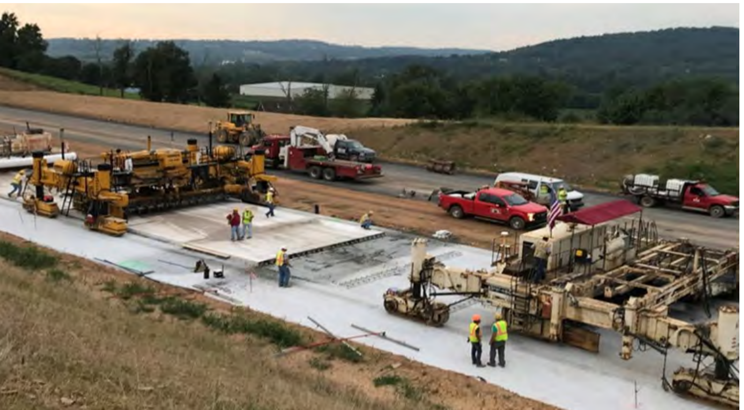
Concrete pavement being placed on the cement-treated permeable base course.
