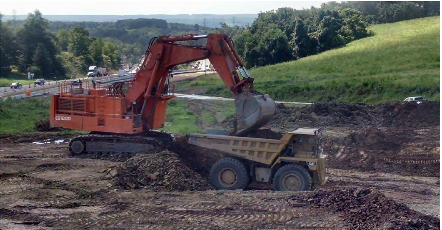
An excavator loading a haul truck near Route 15.
