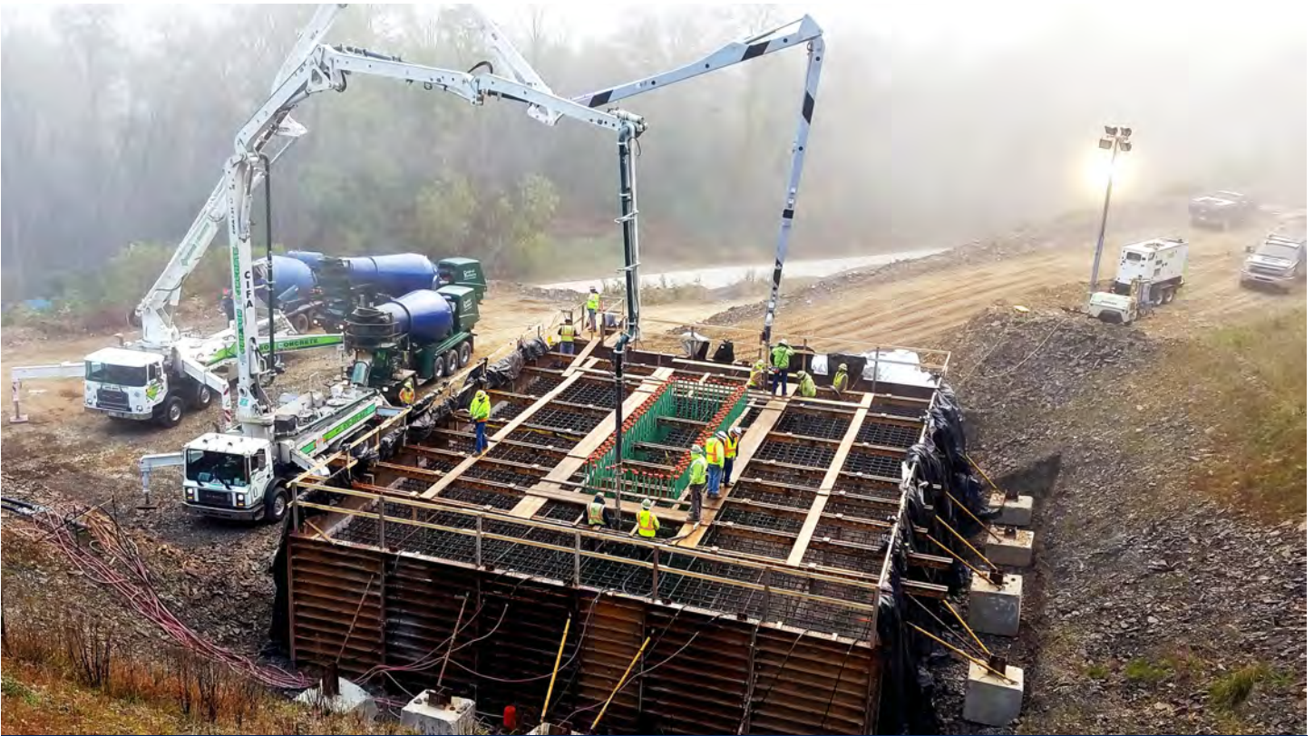
Construction of a land pier foundation.
