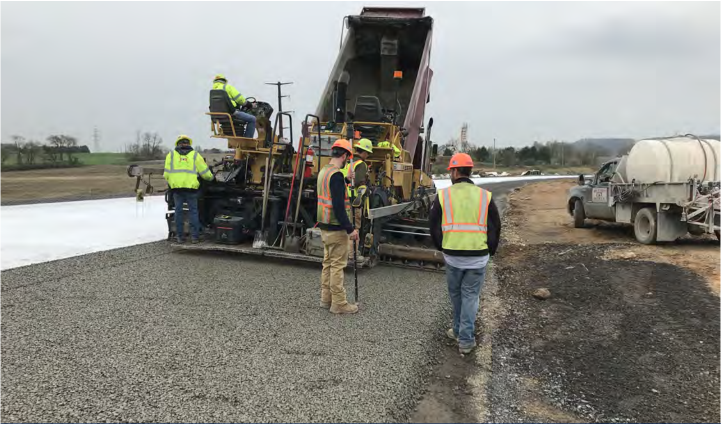
Placement of the cement-treated permeable base course.
