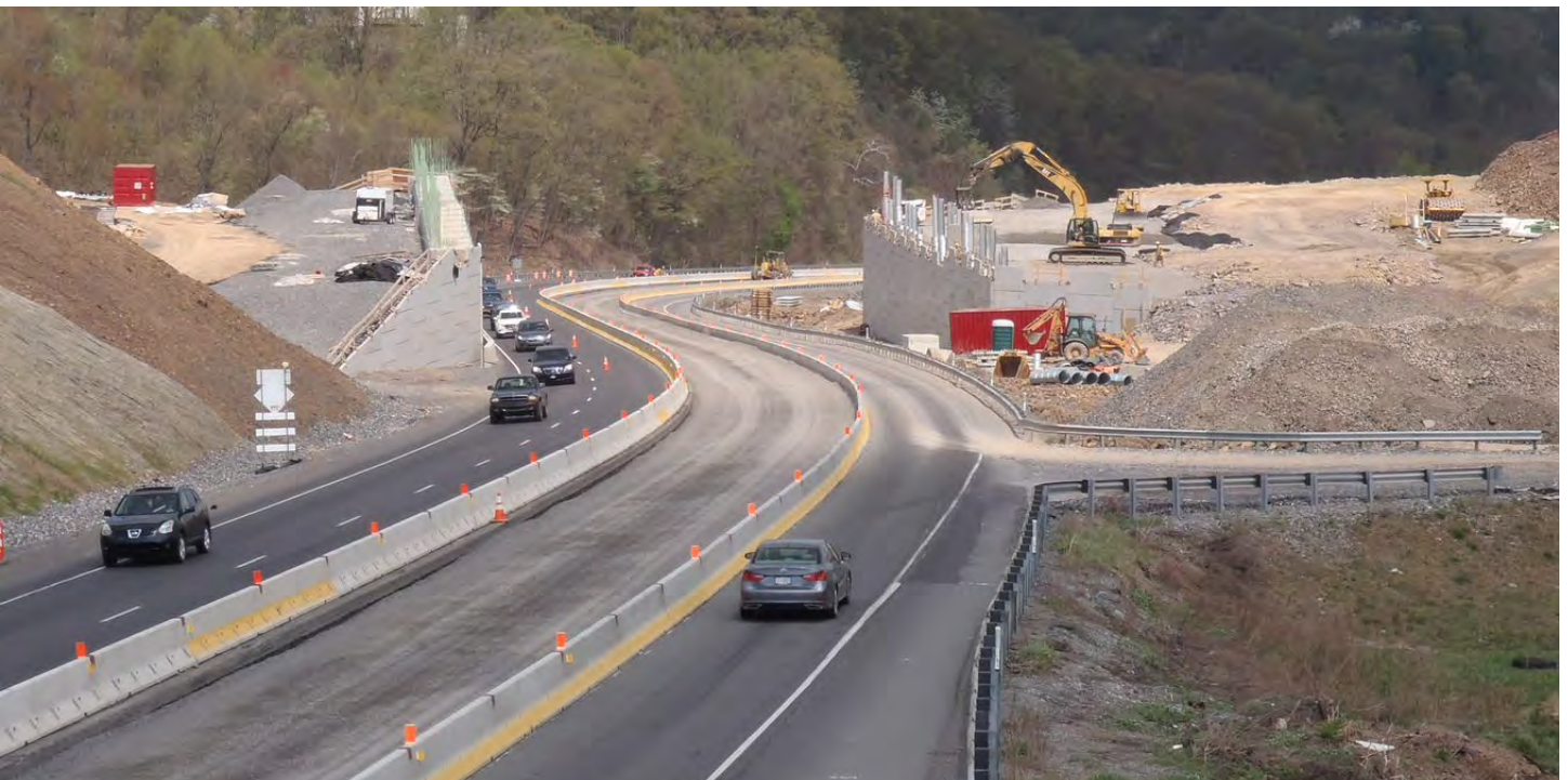
Construction of the bridges over existing Route 15.
