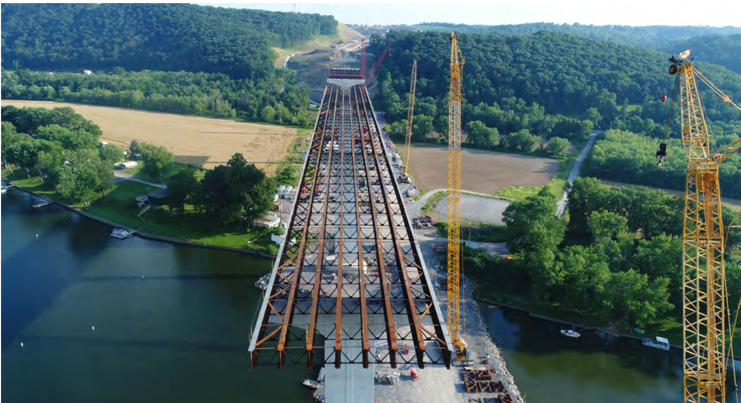
Beams set from the temporary causeway in the river.
