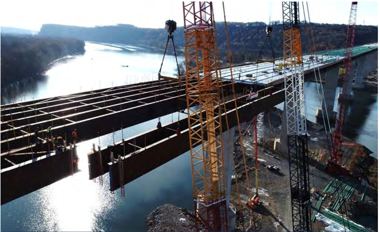
The final beams being set in place.
