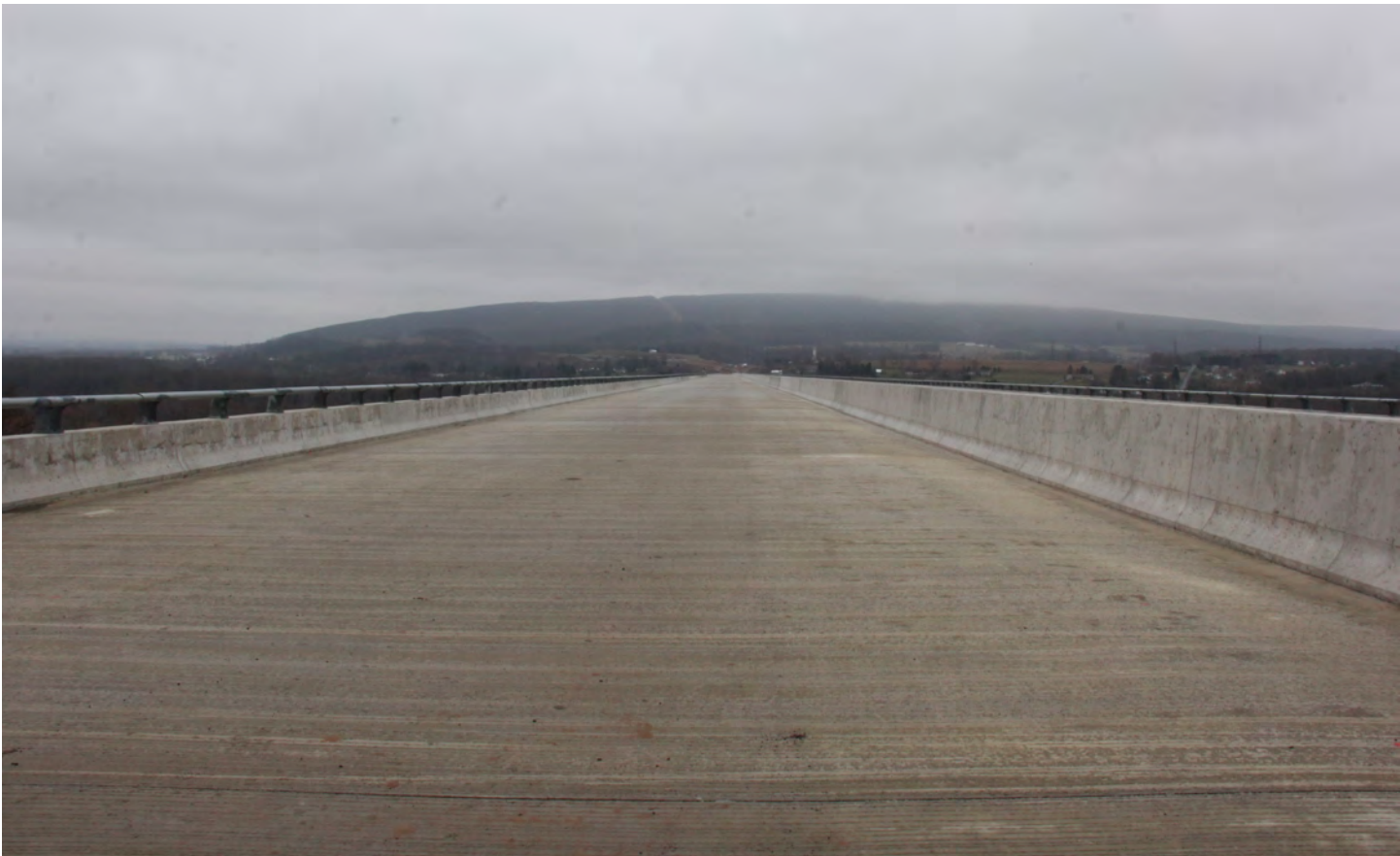
The finished concrete bridge deck, looking north in the southbound lanes.
